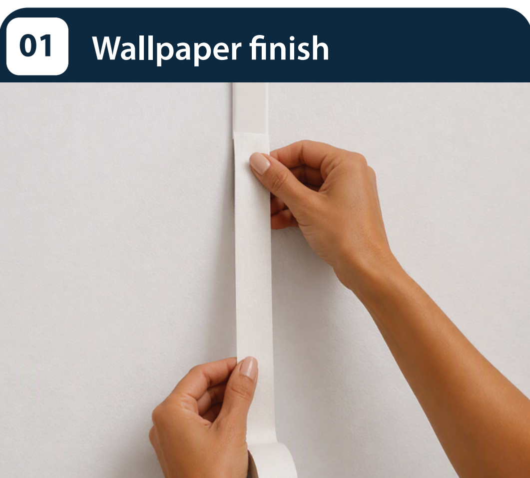
Stick the provided paintable wallpaper roll over the cable.
