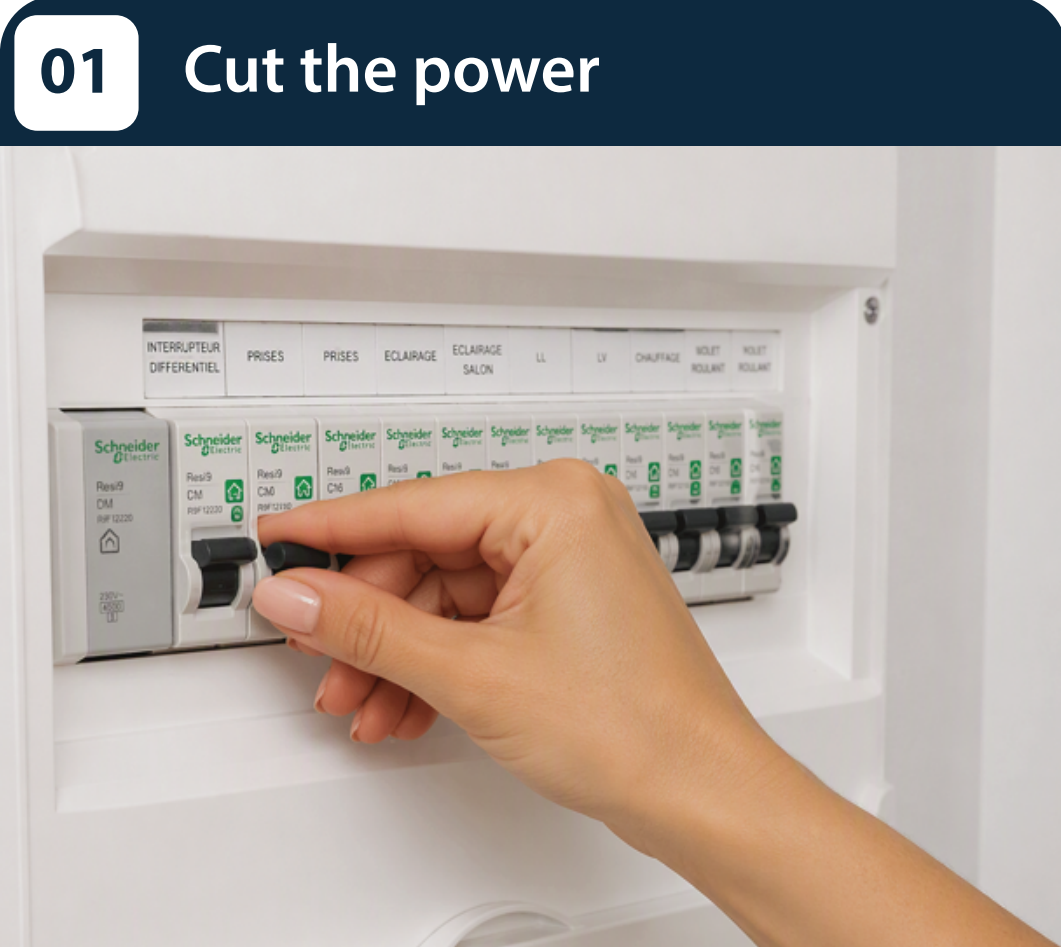
Turn off the power supply and verify the absence of voltage before handling.
